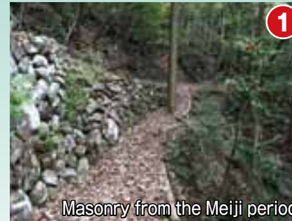
Masonry from the Meiji period Here and there along this road you can see excellent stonework from the Meiji era (1858-1912).
